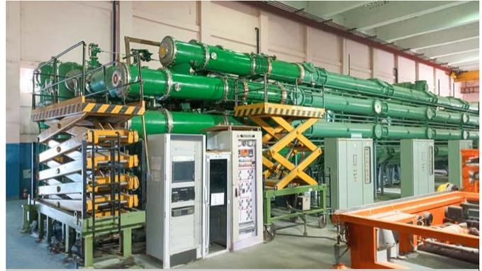
*400kV Gas Insulated Switchgear (GIS) bay at Chamera HEP indigenously developed by BHEL under the Aatmanirbhar Bharat initiative*
