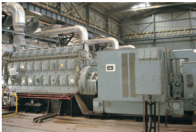
5 MW DG Set for Captive Power Plant at Naval Seabird Project
