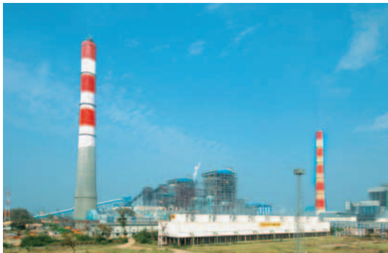
India's largest power station, 3,200 MW Vindhyachal STPS, equipped with 4 BHEL sets of 500 MW each
