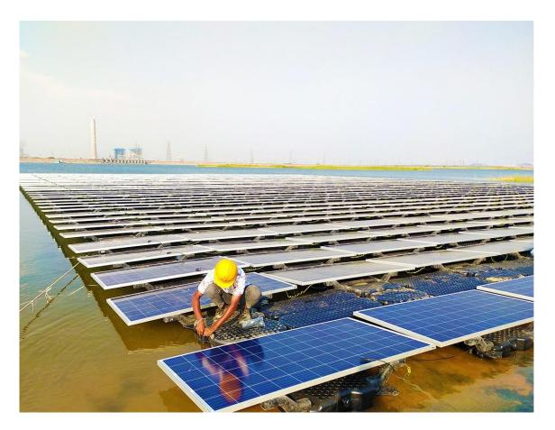
New Delhi, July 7: Bharat Heavy Electricals Limited (BHEL) has successfully commissioned India's largest floating Solar PV plant rated at 100 MW at NTPC Ramagundam in Telangana. The plant is installed across the natural raw water reservoir, saving valuable land resources, and also conserves water by reducing evaporation.
