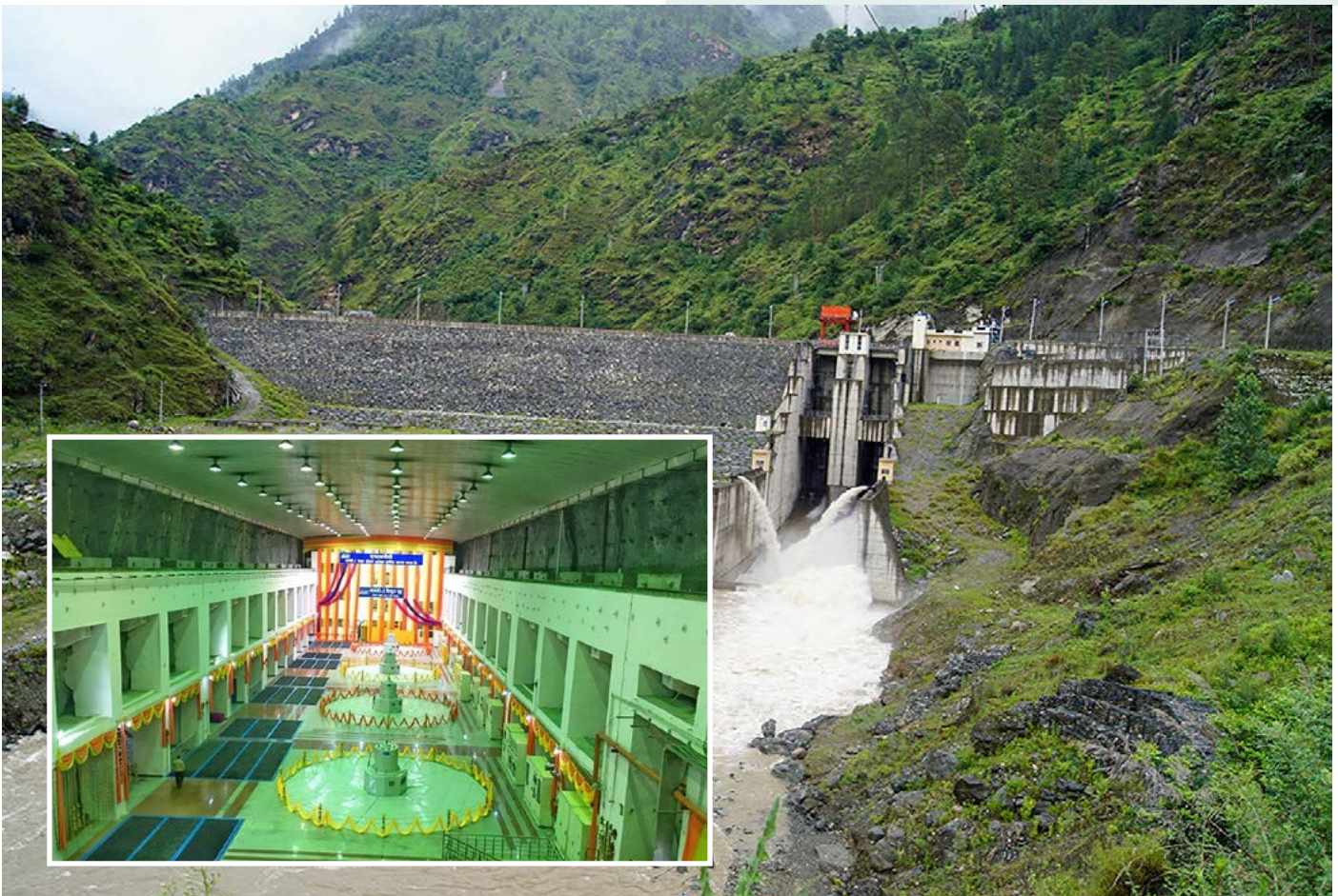
Exterior view of (Inset: Generator floor) 4 x 130 MW Parbati-III HEP, NHPC Ltd. In Himachal Pradesh, India
