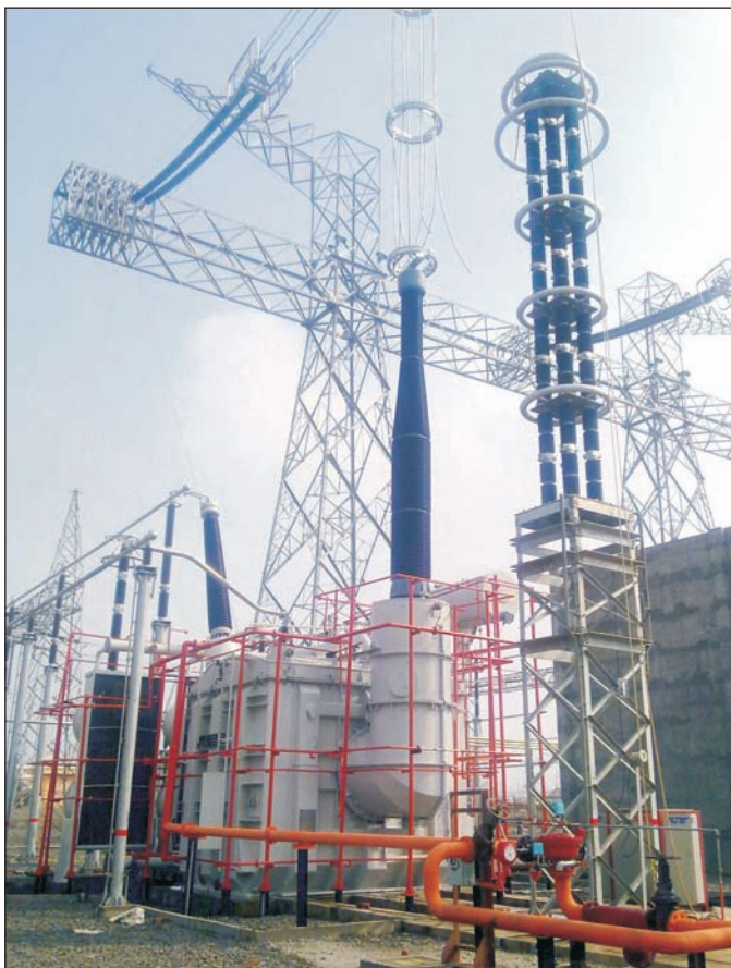
1200 kV Transformer at PGCIL Test Station at Bina
