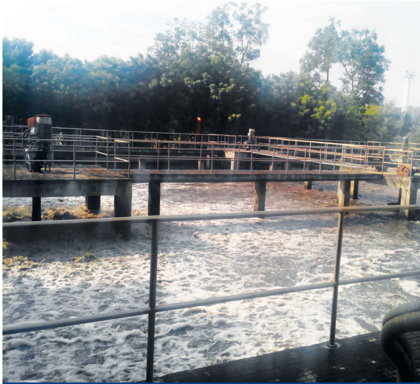
Activated Sludge Process (ASP) based STP at Chennai
