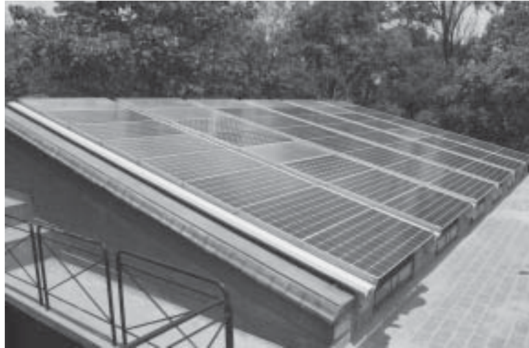
5 KWp integrated photovoltaic system installed at IISc, Bangalore
