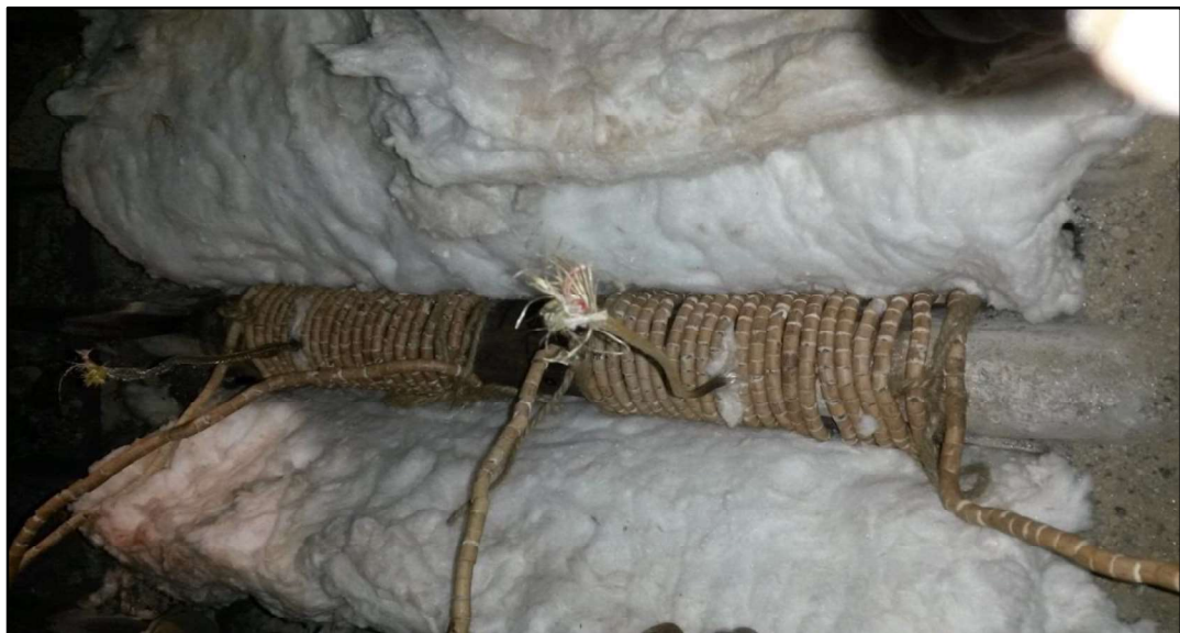
Figure B3.3: Preheating arrangement with thermocouples in place
